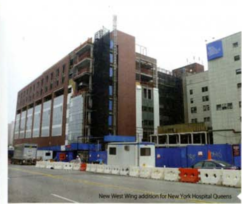
New West Wing addition for New York Hospital Queens
